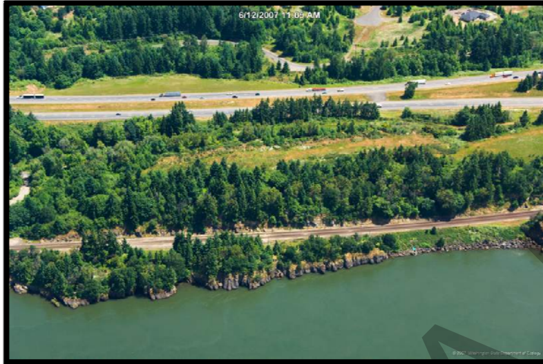
This picture (looking north) shows the rail corridor which runs immediately adjacent to the river.
